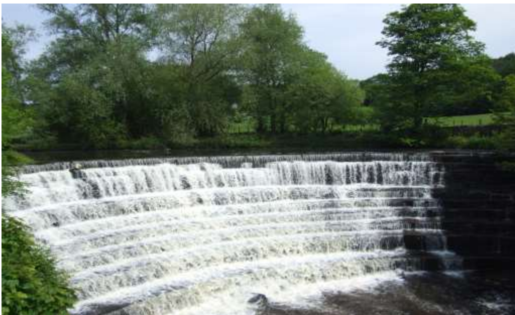
Fig 9 Weir River Etherow Country Park Weir 2018
