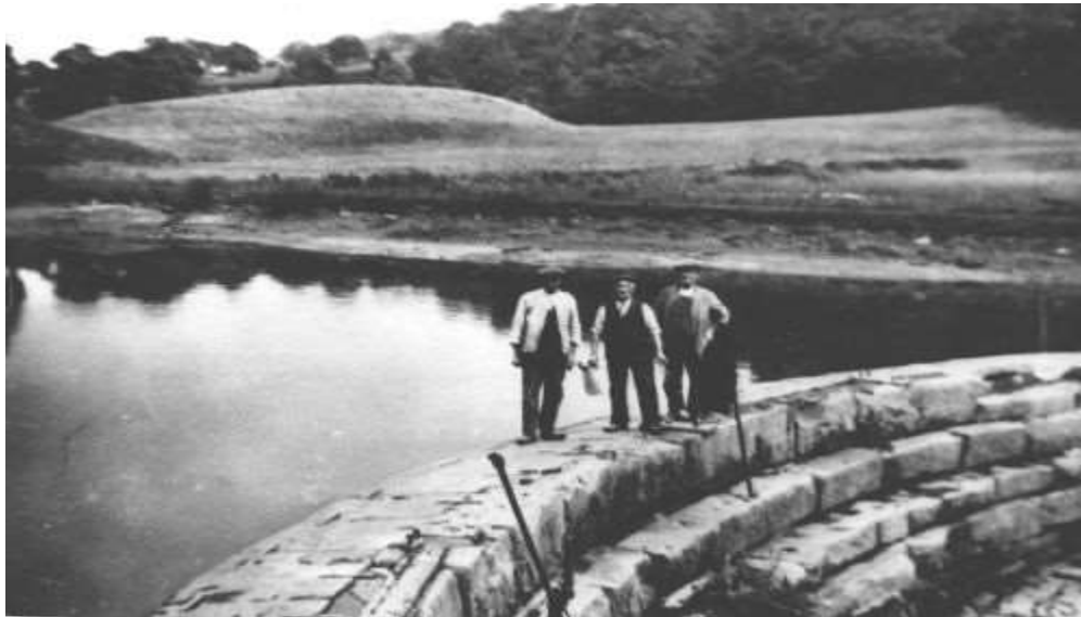
Fig. 8 Construction of Etherow Weir circa 1890
