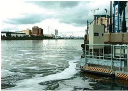
Following comprehensive field trials of suitable oxygenation technology, APEM recommended the installation of a direct oxygenation system. This system has subsequently been successful in elevating dissolved oxygen levels, and thereby improving water quality in the Turning Basin of the MSC, since 2001. APEM have been involved in the management and operation of this system since 2001.
